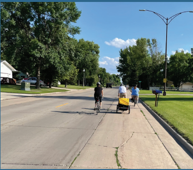
Pavement Conditions – Poor pavement conditions frequently influenced route selection
