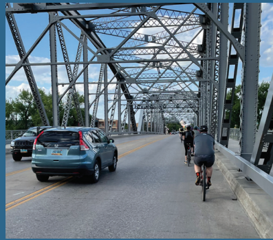
Bridges – The bridges that link Grand Forks and East Grand Forks are a challenge for cyclists.
