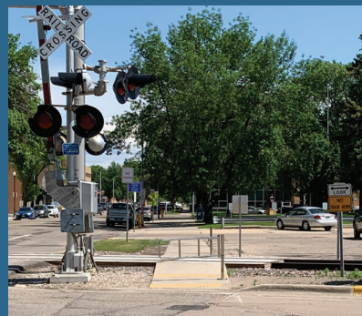
Railroad Crossings – Audit participants stated that rail crossings at Columbia Road and Washington Street are difficult or uncomfortable to use.
